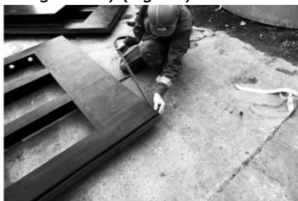
Fig. 1.7 Assembly of gaskets on the weirs
