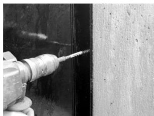
Fig.1.11. Openin drilling for anchors connecting weirs with the tank
