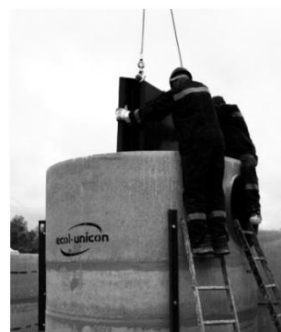
Fig.1.8. Placing the weirs inside the separator tank
