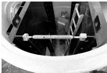
Fig.1.9. Inner weirs before connecting it with the separator tank
